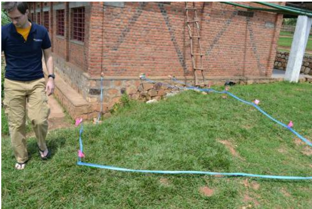
Dryer building layout in blue tape for review with orphanage director, orchard project manager, and building construction lead.
